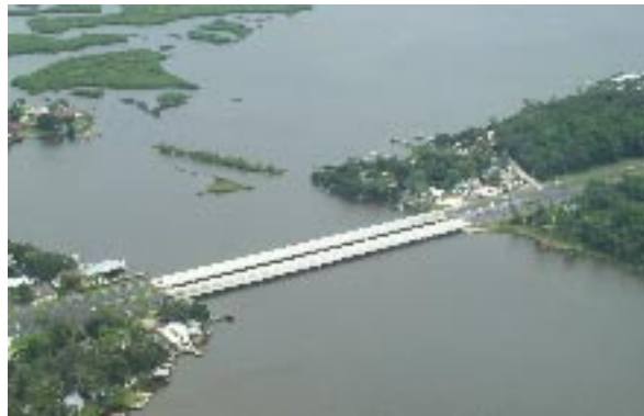
Fig. 2. Rose Bay Bridge.
