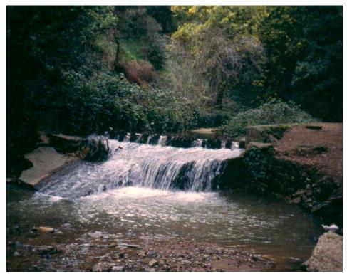
Failing concrete check dam before project construction, looking in upstream direction. Photo: Drew Goetting (WRI), 2000
