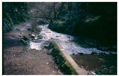
Channel bank erosion at failing concrete check dam before project construction, looking in downstream direction. Photo: Drew Goetting (WRI), 2000
