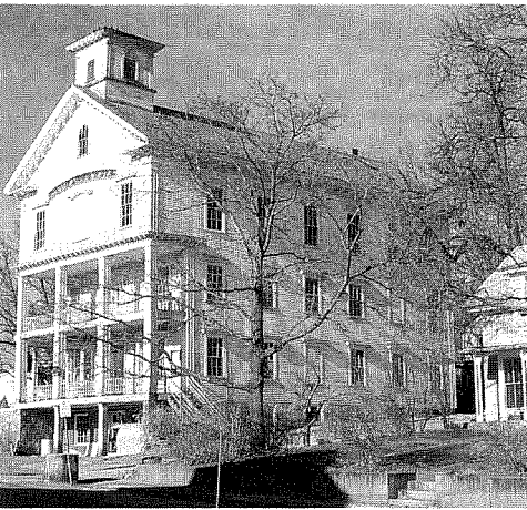
A typical community building.
