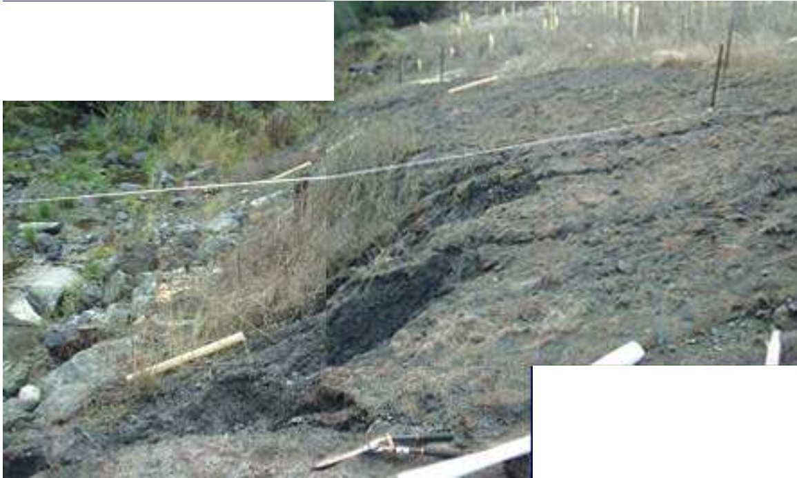
FIGURE 18. View of north bank of Area I. Erosion at transition from stream bank to regraded hillslope is evident. Photo taken by Alicia Gilbreath on November 3, 2005.
