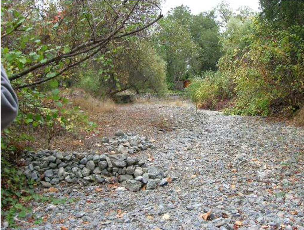
FIGURE 7. Rocks piled near left bank downstream of Crocker Creek Dam removal site. Looking downstream. Photo taken by Maureen Downing-Kunz on November 3, 2005.
