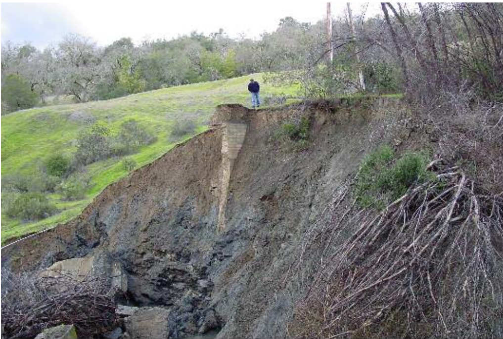
FIGURE 2. View of the north abutment (Area I), after the '95 and '97 Crocker Creek dam failures in 2002, prior to restoration. Unknown photographer, image courtesy of SCWA.
