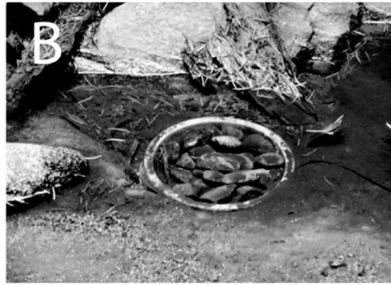
Fig. 2.4. An example of the sediment traps before (a) and after (b) stream crossing-reconstruction.
