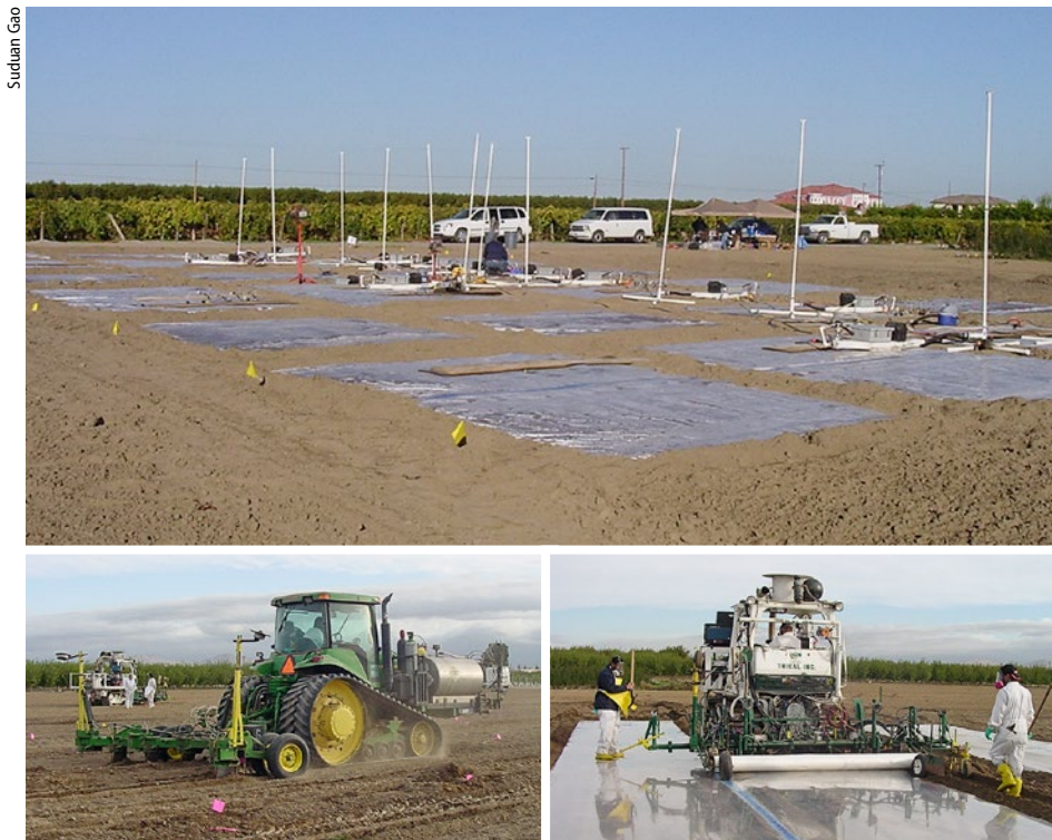
Researchers used dynamic flux chamber equipment, top , to measure fumigant emissions throughout the fall 2009 trial period and 24 hours after tarp cutting. Bottom left , fumigant injection; bottom right , plastic tarp installment at Parlier, Fresno County.
