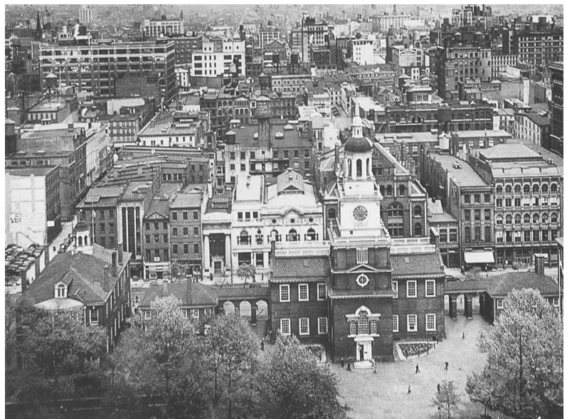
Independence Hall, view to north, 1952 Courtesy Independence National Historical Park
