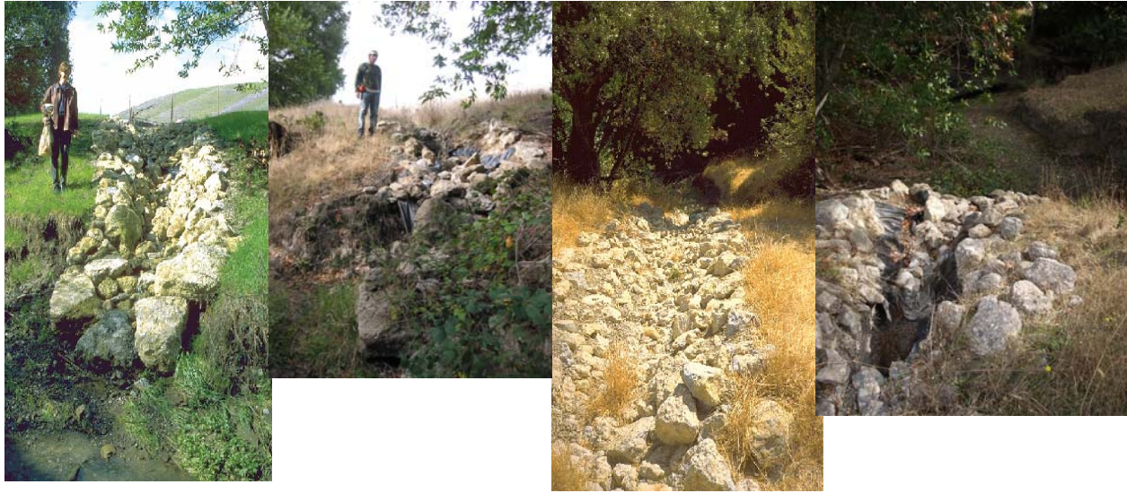
Figure 13: Structure 16 storm drain
