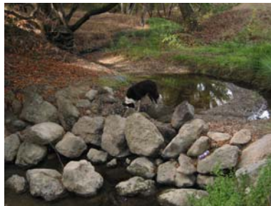
Figure 9:GC2 from downstream appears stable
