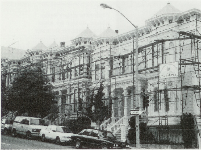
San Francisco's Victorian rowhouse, a quintessential type of thin building, has demonstrated its adaptability over the years. (Christie Johnson Coffin)
