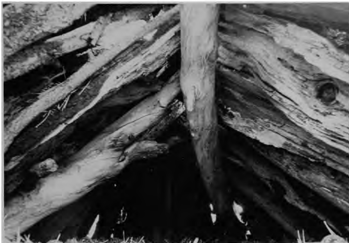
Fig. 5. Ceiling detail of piagi storage structure shown in Figure 4.
