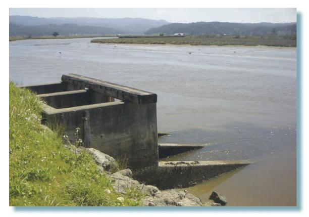
**Figure 25.** Tide gate separating Eureka Slough, Humboldt Bay, Humboldt County, California, and the drainage ditch that parallels California State Highway 101. Eureka Slough is in the background.
