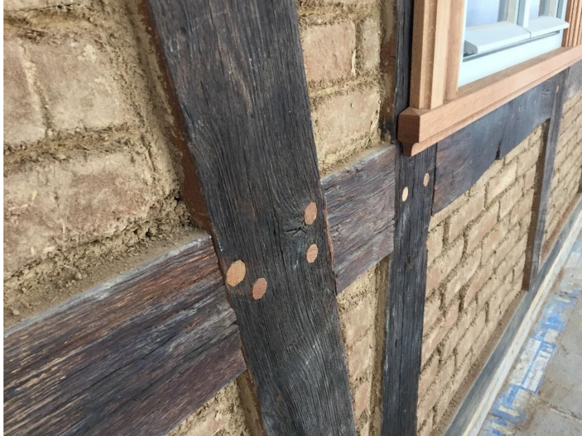
Fig. 3 Half-timber construction on the "Hof zum Rebstock" in the Dom/Römer reconstruction project in Frankfurt am Main (2016).
