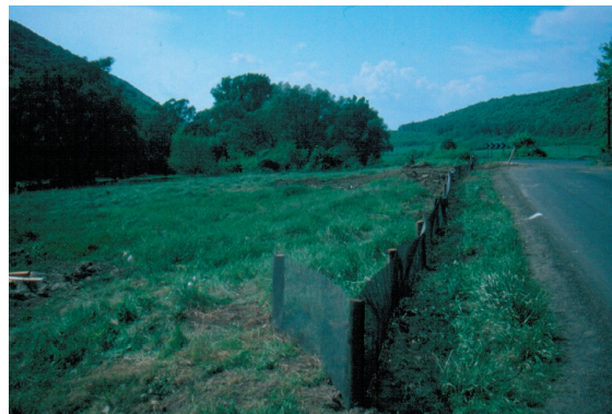
Photo 15. The end of the fence is turned back to prevent amphibians from getting onto road.
