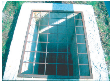
Photo 18. Diagonal light shaft in the median of a motorway.
