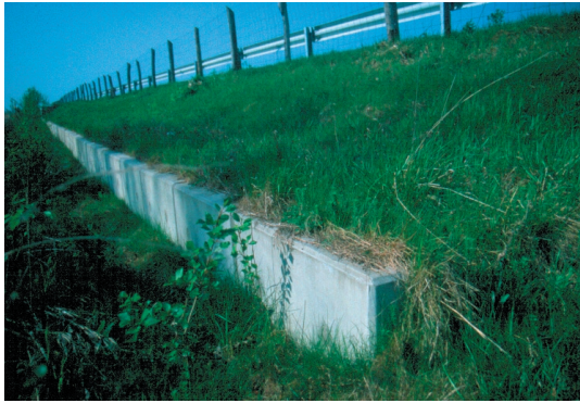
Photo 11. Concrete fence on motorway, Hungary.
