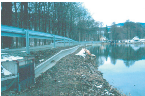
Photo 5. Modern amphibian mitigation measure at Kudowa Zdroj, Poland.
