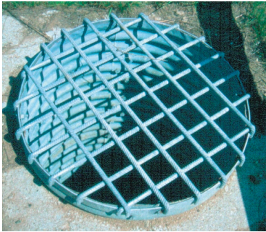
Photo 16. Circular light shaft in the median of a motorway.
