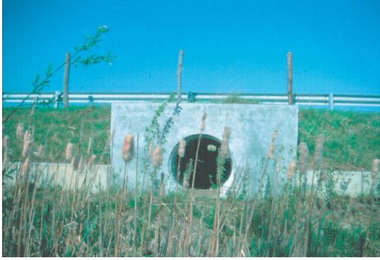
Photo 7. Circular tunnel opening and concrete fence.
