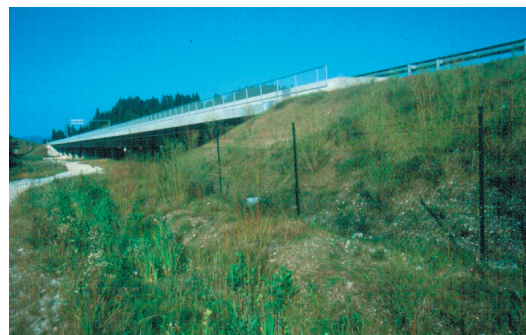
Photo 6. Modified viaduct for game and amphibians at Domzale, Slovenia.
