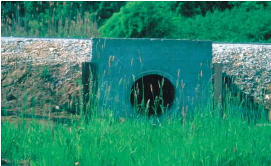
Photo 9. Circular tunnel opening, plastic mesh fence fixed by wooden pole.
