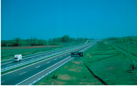
Photo 1. Amphibian measure with 45 degree angle fence arrangement along the M3 motorway, Hungary.
