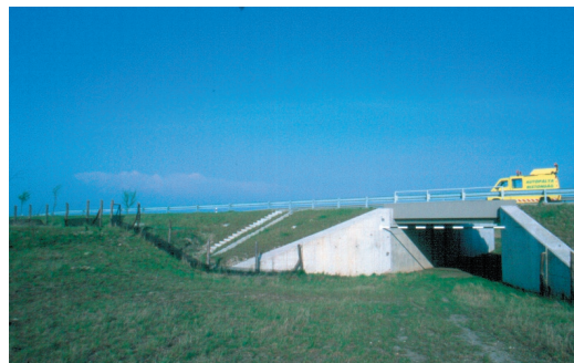
Photo 4. Game passage with amphibian fence under the M15 road, Hungary.
