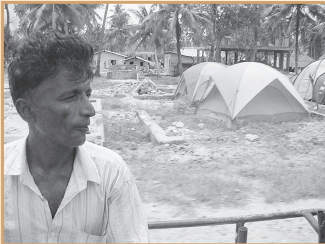
In a village between Pereliya and Hikkaduwa, Sri Lanka tent shelters sit on top of wave washed foundations more than four months after the tsunami
