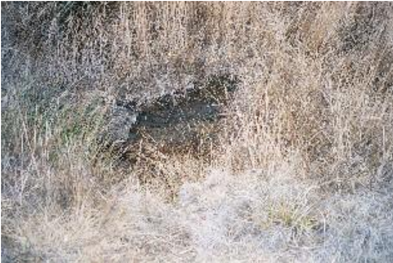
Figure 6. An exposed gully North Tributary #2.
