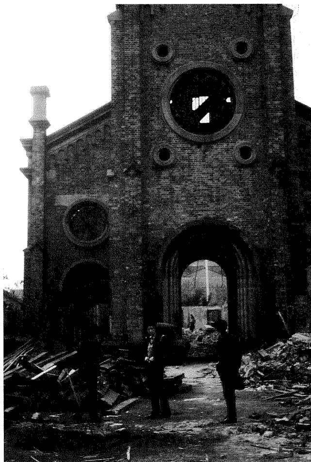
During the Cultural Revolution, many Western-style buildings, such as godowns and churches, were ransacked. The Church of Our Lady, built in 1926, was demolished in 1988.
