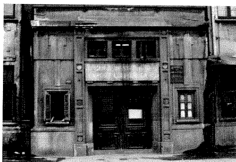
The former headquarters of the China Import and Export Company was abandoned during the Cultural Revolution.
