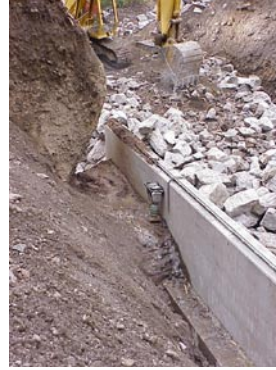
Fig. 11. Machine Labor – 4 day to place 600 CY.
