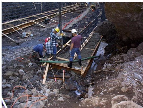
Fig. 6. Concrete is being placed to seal off water at upstream end of form first.
