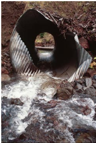
Fig. 1. Possible confusing survey areas - folded pipe invert, high relief boulder stream.
