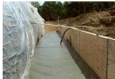
Fig. 8. Placing flowing mortar bedding. Photos courtesy of Contech CPI
