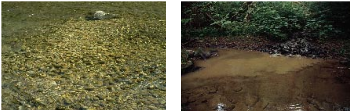
Fig. 4. Construction-generated sediment effects on streambed, before and after excavation.
