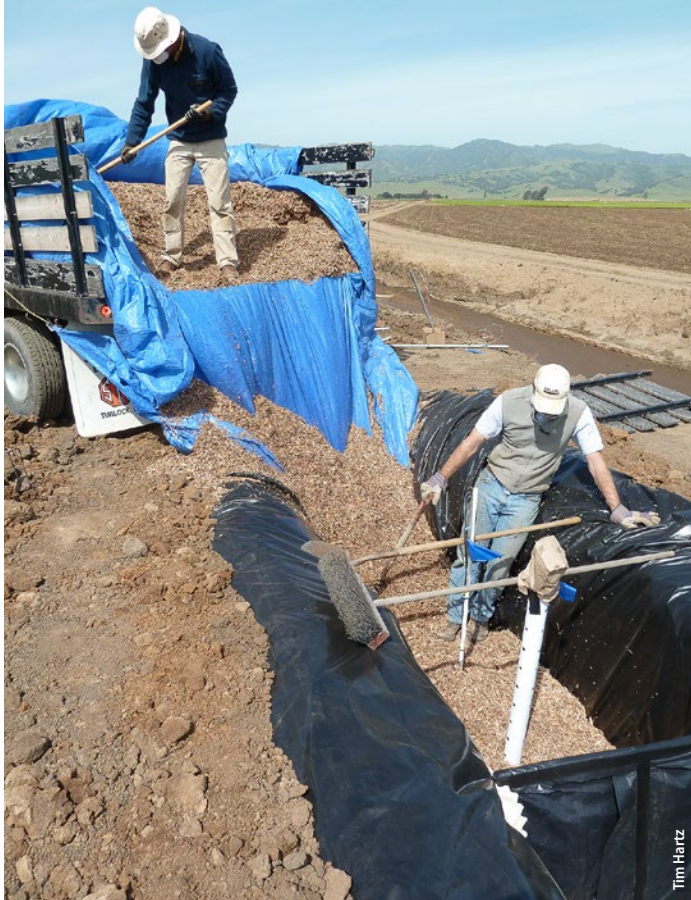
Denitrification bioreactor being filled with wood chips.
