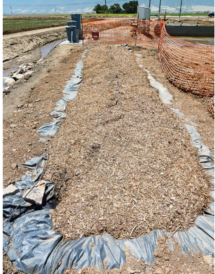
Completed denitrification bioreactor.
