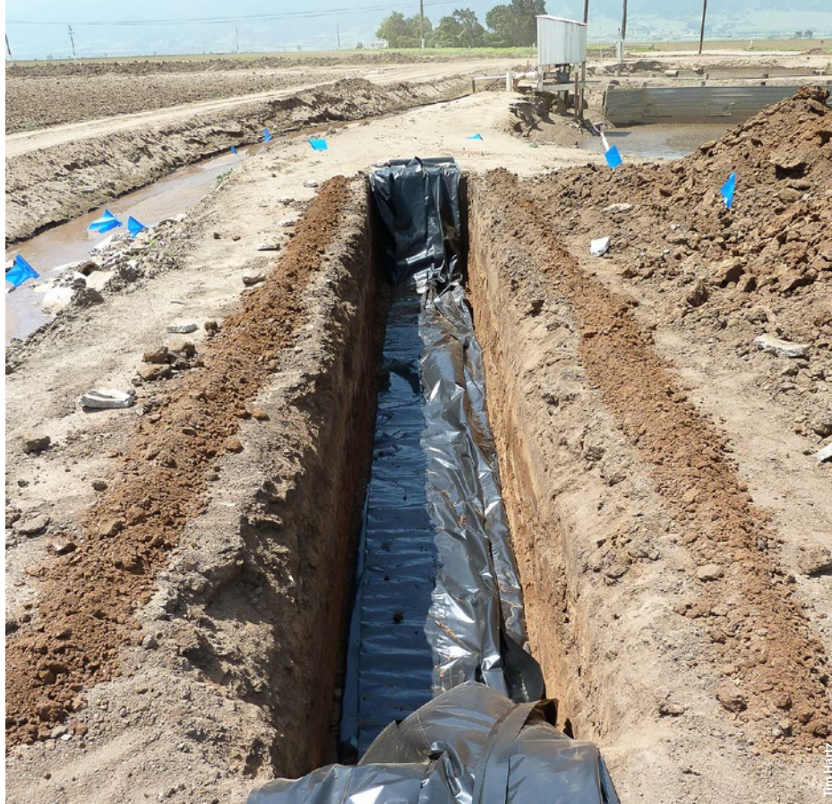
The denitrification bioreactor was dug with a backhoe and fitted with a polyethylene liner.
