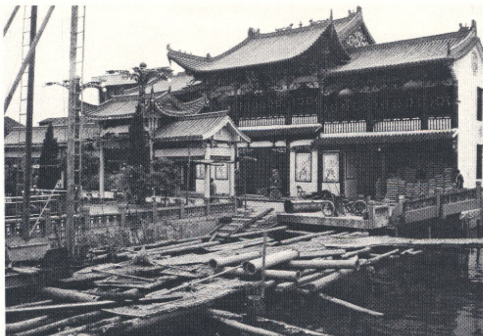
Figure 4. Tianxian Gong (Palace of the heavenly immortal) after renovation and expansion (photo by author, 1998).
