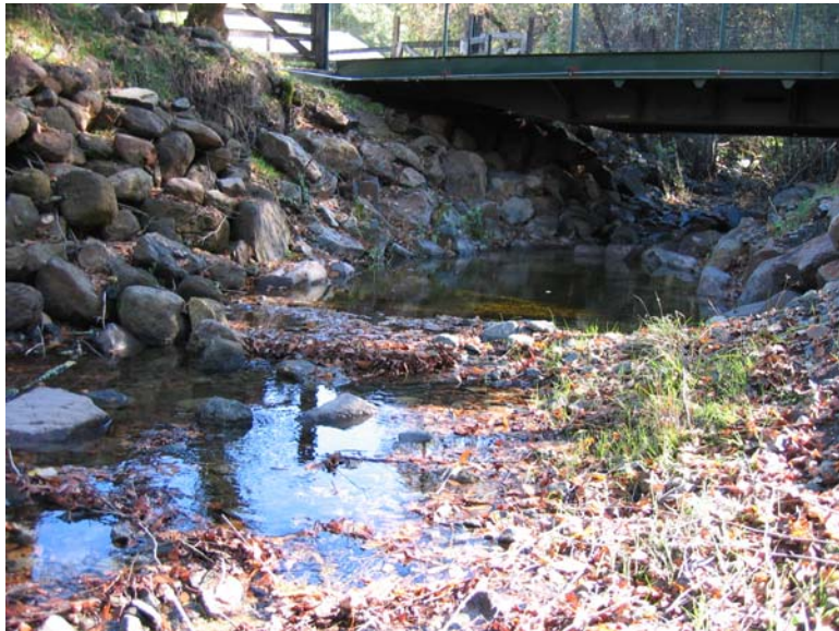
November 2007- pools below bridge
