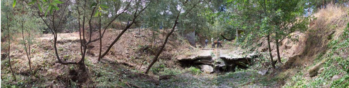
October 2004 During Demolition, Photo by Lara Hadhazy, Napa County RCD
