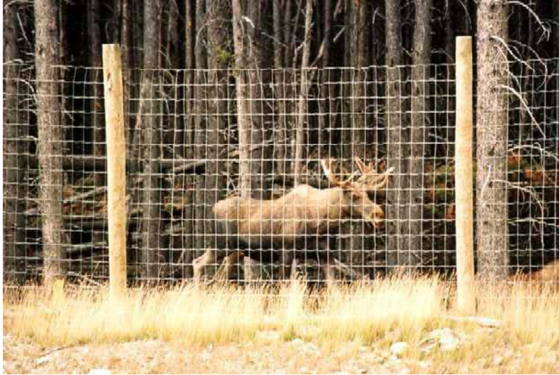
Figure 16. Wildlife exclusion fencing designed for moose
