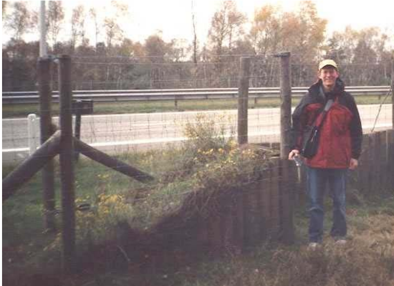
Figure 11. Earthen ramp designed for deer in Belgium
