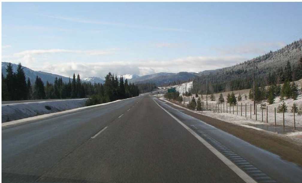
Figure 15. Wildlife exclusion fencing on Coquihalla Highway
