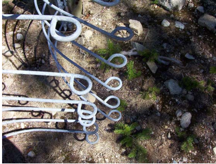
Figure 6. One-way gate with “looped” tynes
