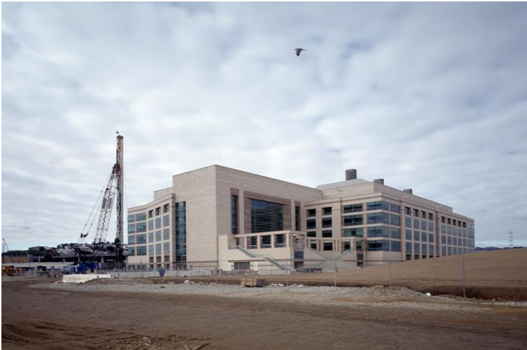
Figure 10-10. The initial UCSF building at Mission Bay (Genentech Hall) under construction, 2002 205
