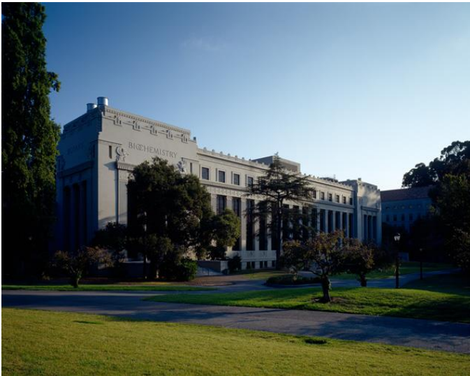
Figure 12-1. The Valley Life Sciences Building, with Life Sciences Annex in the shadow to its right 65
