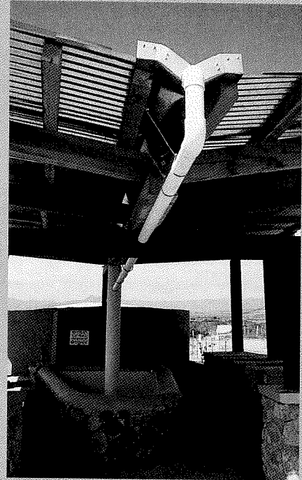
Santa Ursula public lavandara , detail of roof and water conveyance system. Photo: Daniel Winterbottom.
