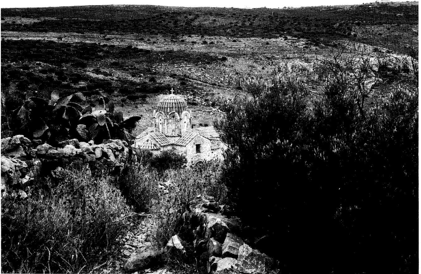
Episkopí (c. twelfth century). Stavri, Laconia. The approach to this church in the Mani, seemingly perched in the hollow of a hill, presents a view of the restored cupola, apse and north side of the transept. Beyond is the Bay of Mésapos and the peninsula of Tigáni.
