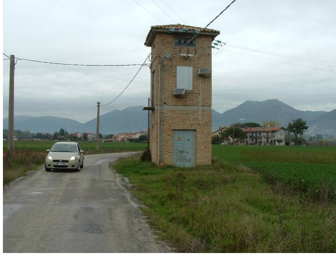
Figure 2.11. ENEL electrical substation housing a recording instrument in Gubbio-Piana site (Umbria)
