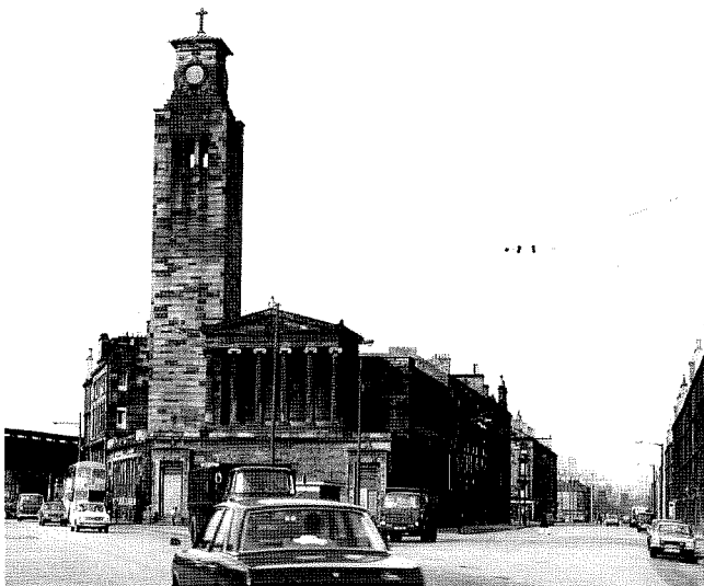
Above: Caledonia Road United Presbyterian Church, photographed by author after its gutting by fire and touched up to resemble the form of its earlier urban appearance. Right: Caledonia Road church sits at a point where two grids meet. Thomson used nearby tenements, which he also designed, to help knit the church into the city.
