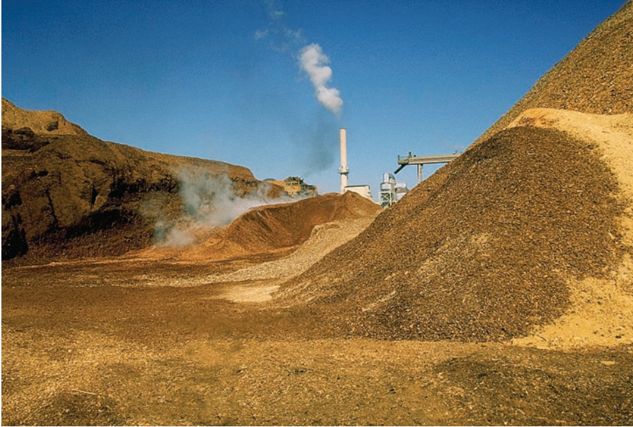
An estimated 14 million dry tons of forestry residues could be sustainably processed in California each year for energy. Above, large piles of wood chips are mixed together before being burned in the distant power plant.
