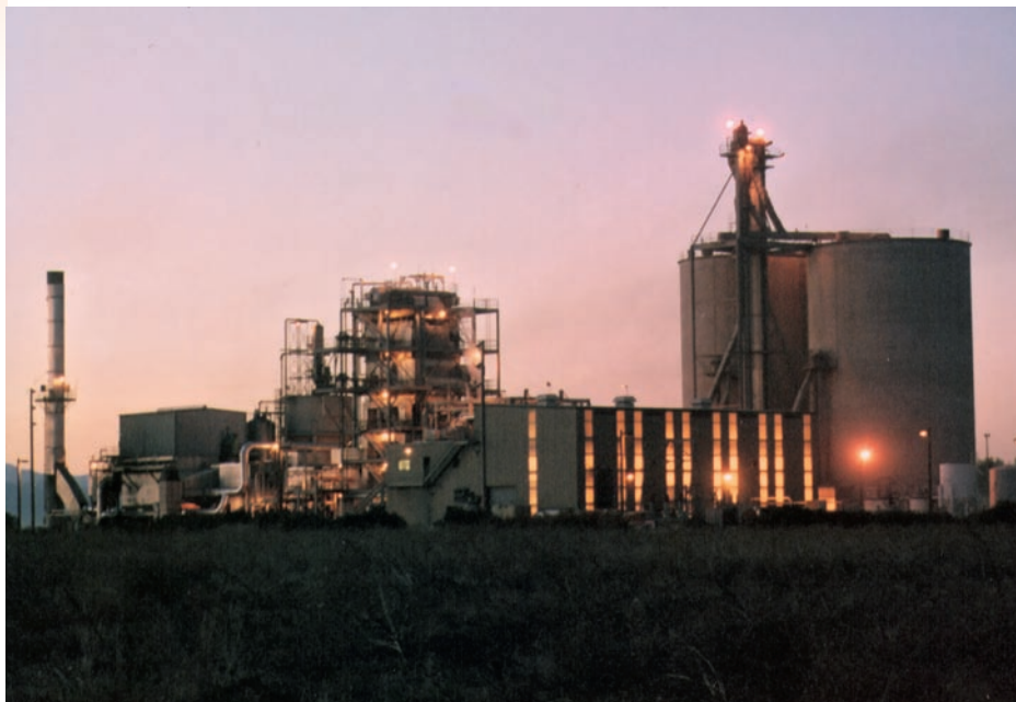
Wadham Energy power plant in Colusa County near Williams generates 26.5 megawatts of electricity from rice hulls, enough to power about 22,000 homes. The plant is one of about 30 operating in California that generate electricity from solid biomass.
