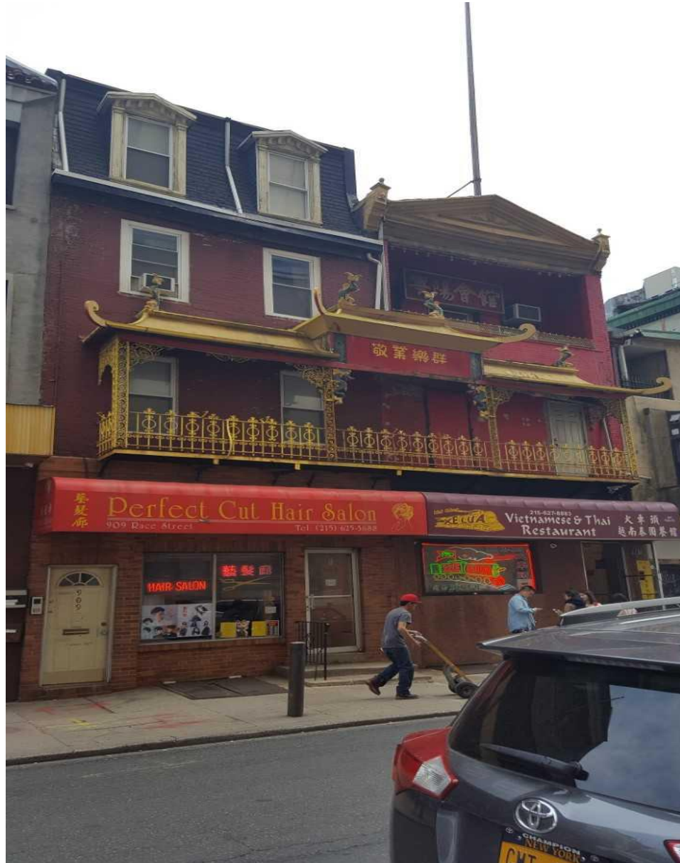
Fig. 9. Interplay of fire escapes, balconies, and roof in Philadelphia Chinatown, Race Street, 2018. Note contrast of commercial entries and doors to upper floors. Photo credit: G. McDonogh and C. H-Y. Wong.
