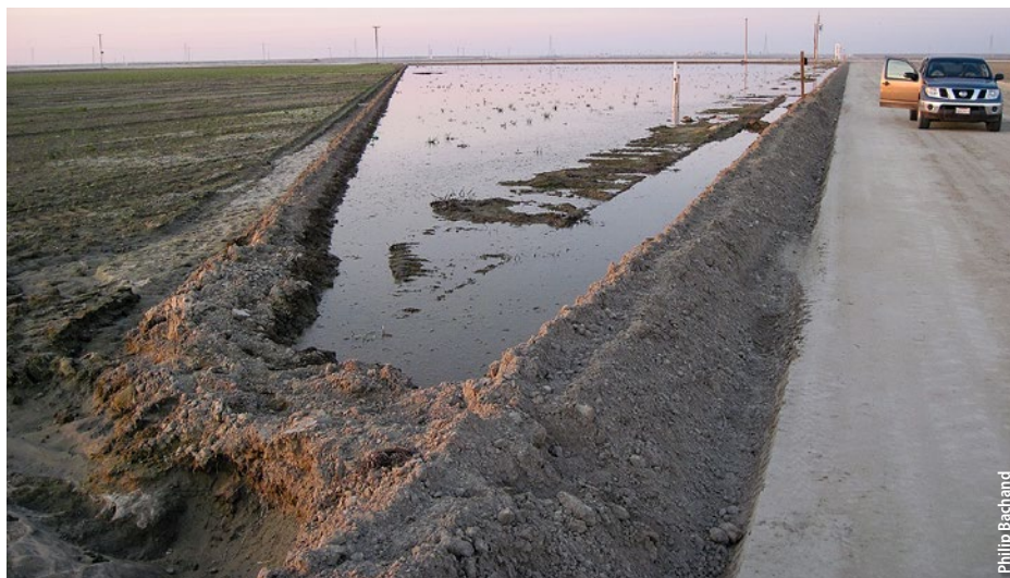
Wintertime modifications to tomato field to manage water were similar to rice checks to enable capture and infiltration of flood flows. Modifications included cutting small check berms to accommodate field gradients and installing low cost flashboard risers to manage water flow and elevations.
