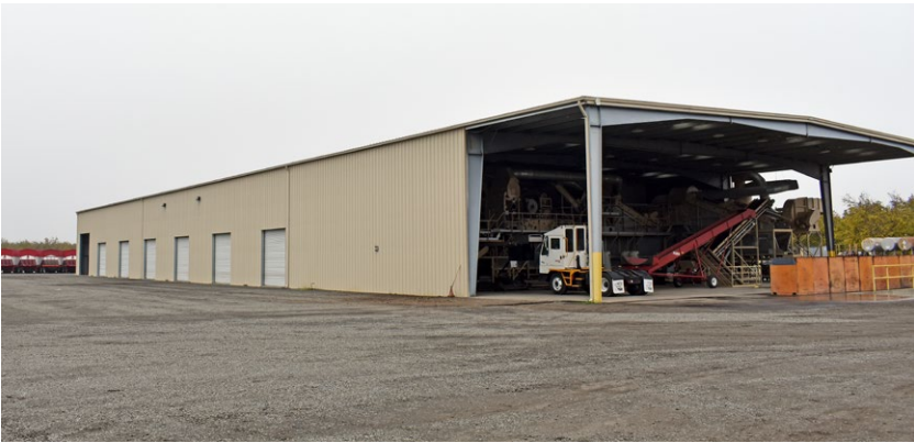
Exterior view of the Fedora Farms, Inc., walnut processing and drying facility. The building contains hulling, cleaning, and material-handling equipment used to prepare walnuts for in-bin drying. The doors along the lateral side are opened during the drying season to intake outdoor air. Photo: A. Dien and I.R. Donis-González.
