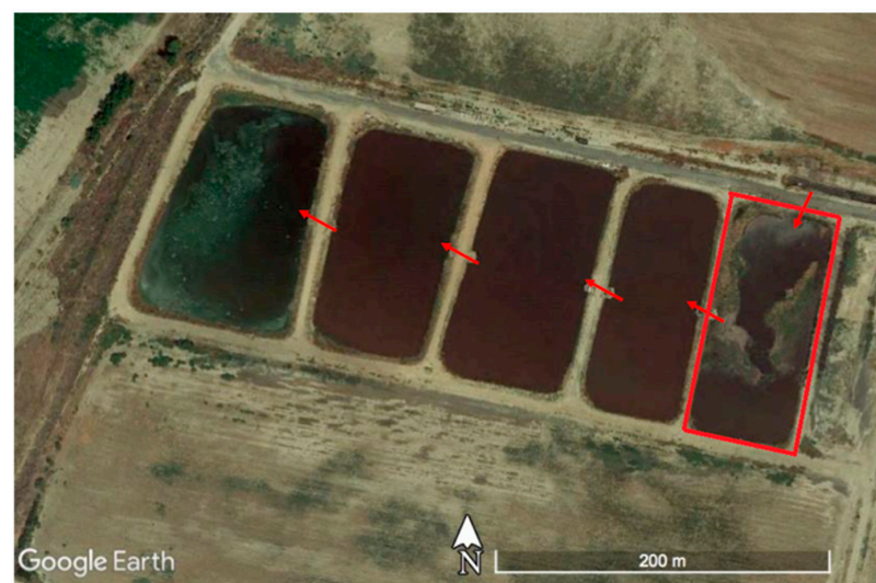
Figure 7. Aerial view of the manure lagoon complex at the southern California dairy. Red arrows show the flow of the manure.
