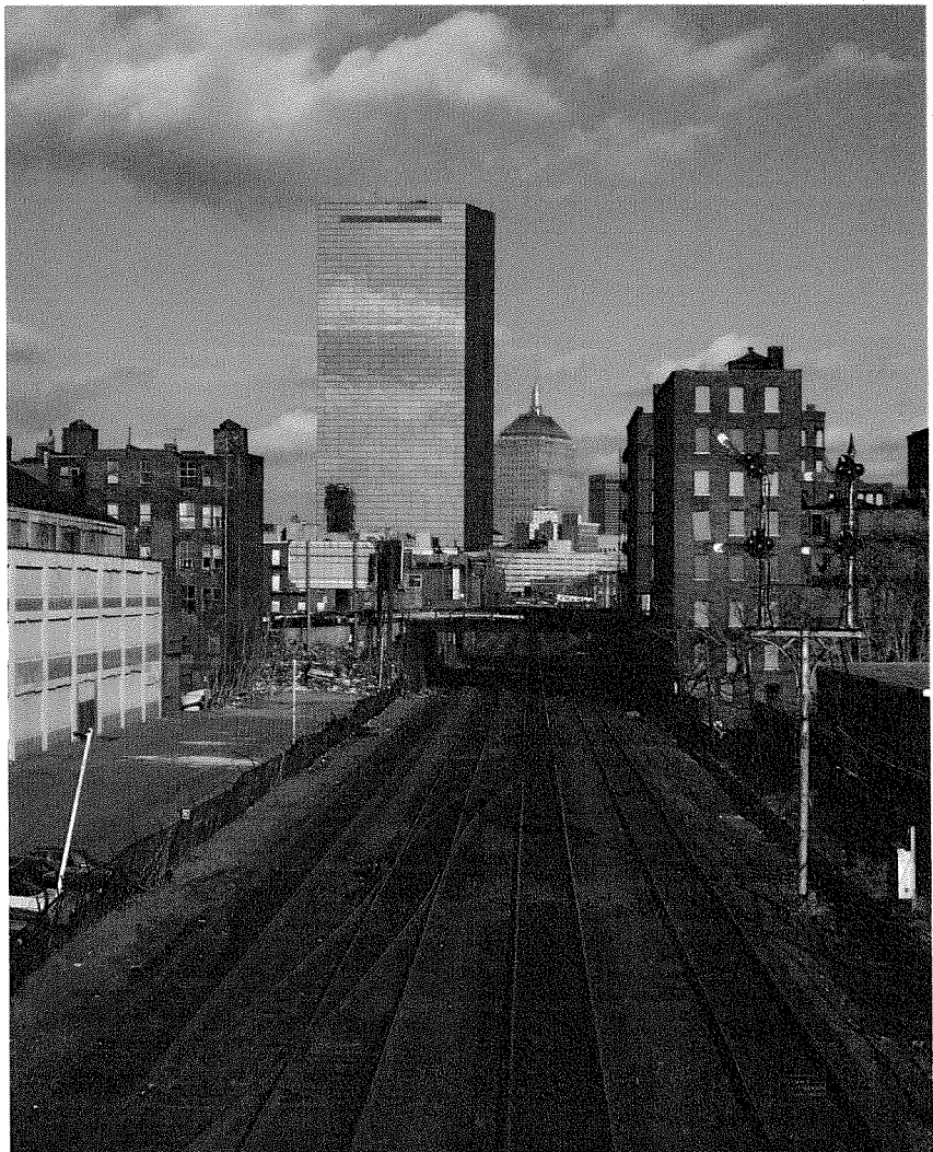
Before the Park, the railroad corridor divided Back Bay from the South End. Photo courtesy Monica and Gary
