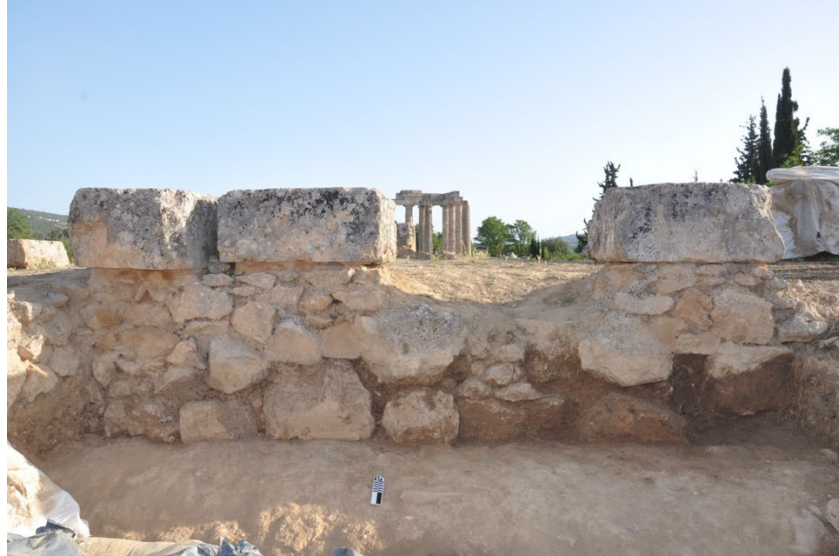
Figure 2. Basilica, Room 3, North wall after cleaning
