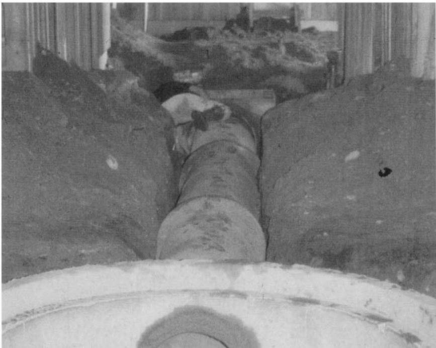
PHOTO 6. Installation of air inflow pipe to fire pit
