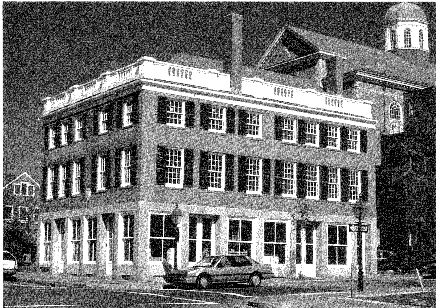
Even after this building was nearly destroyed in an explosion, New Bedford preservationists fought to keep it standing and to rebuild it.
