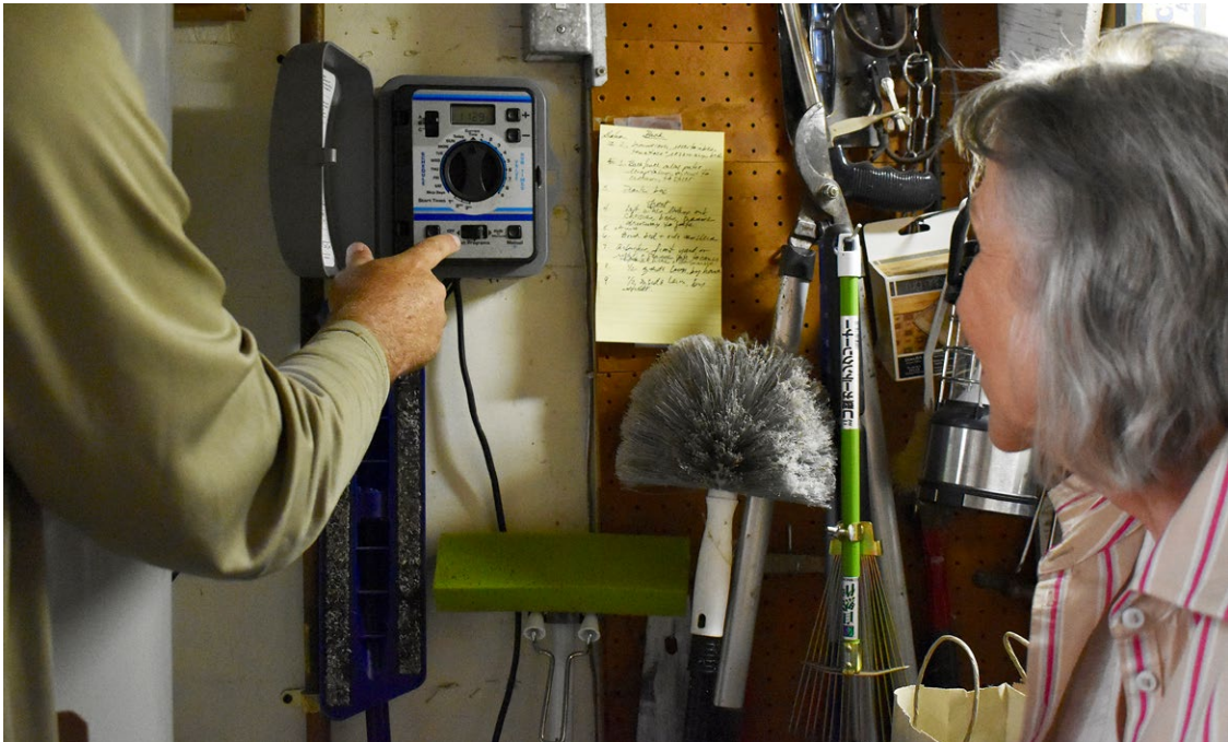
Irrigation frequency and run times are reviewed for each planting zone at the sprinkler irrigation controller. Photo: Rebecca Ryan.
