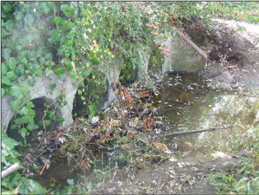
Figure 20: Downstream end of project reach
