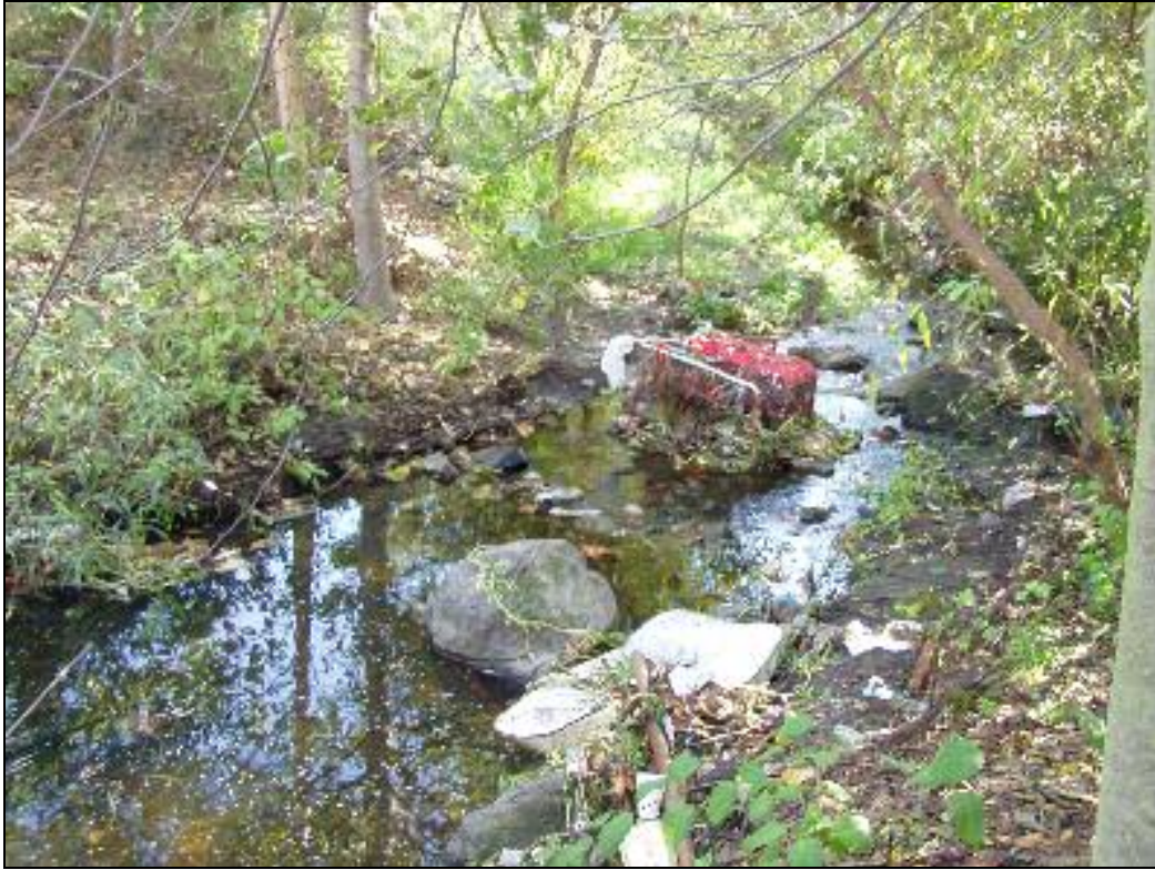
Figure 15: 50 ft from upstream culvert (looking downstream)
